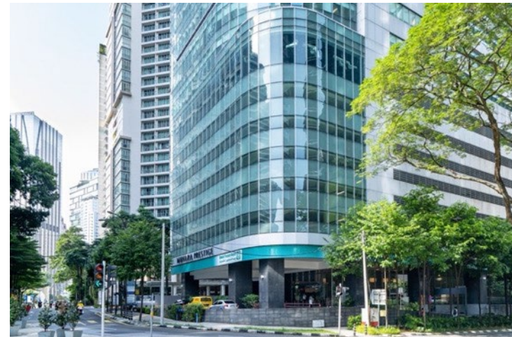
Kintone Southeast Asia Sdn. Bhd. Office building
